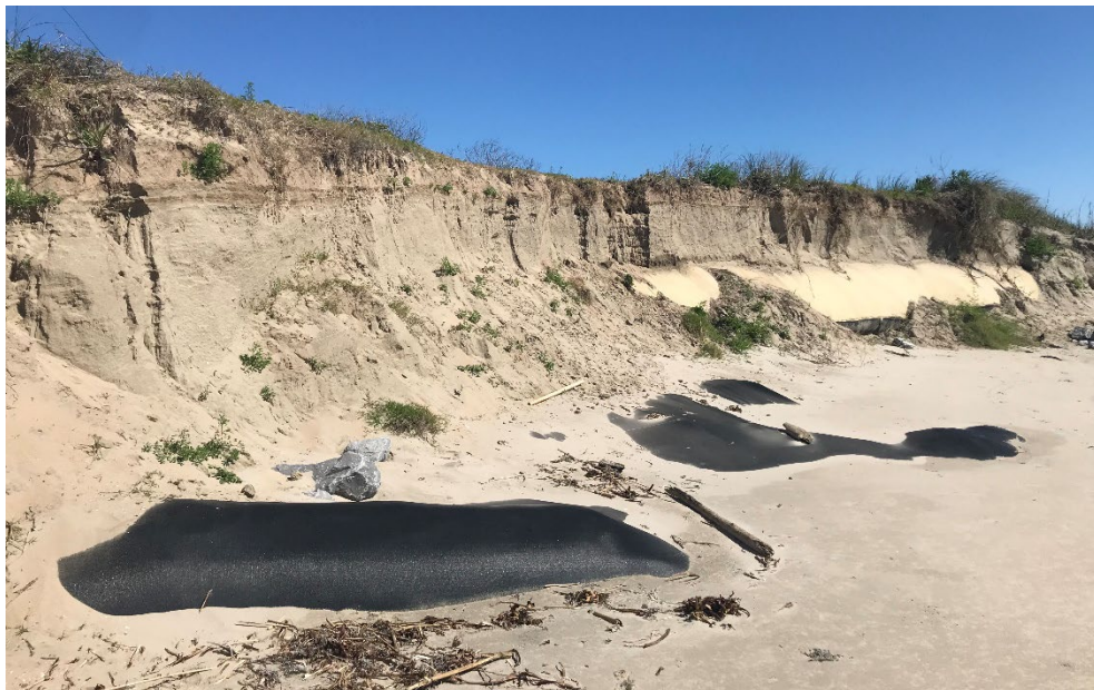
Figure B8: Exposed Geotube
